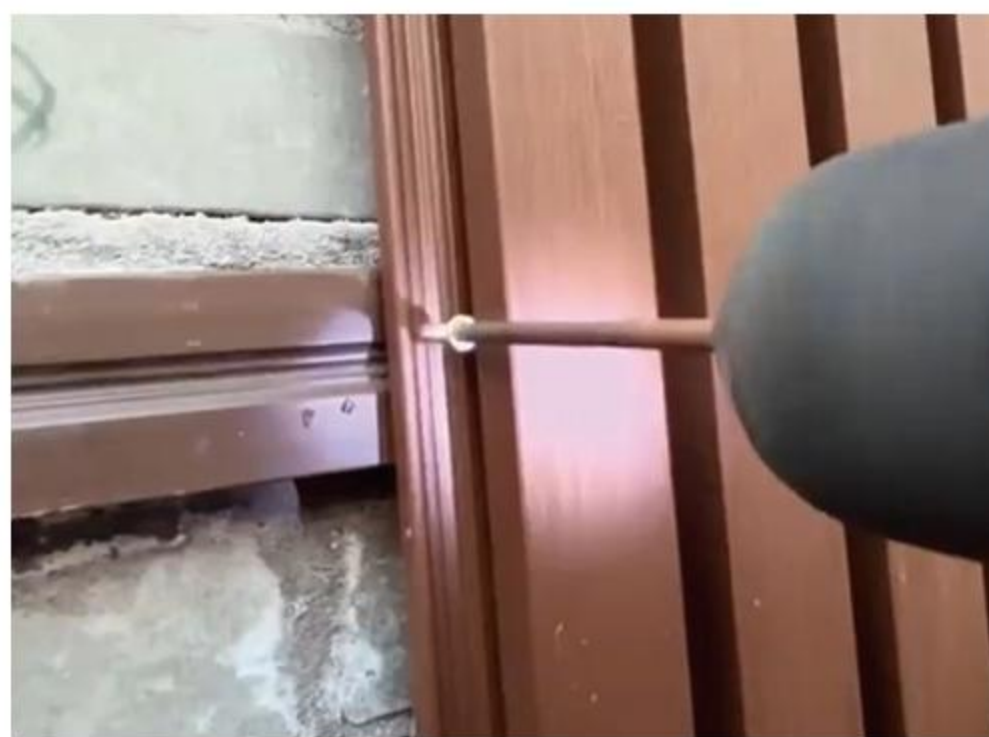
◦ Step 2 Secure the product to the studs.
