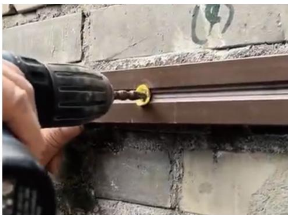
◦ Step 1 Fix the studs to the wall.
