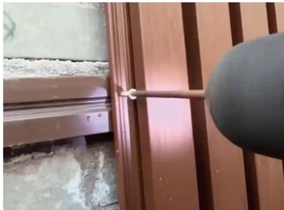
◦ Step 2 Secure the product to the studs.
