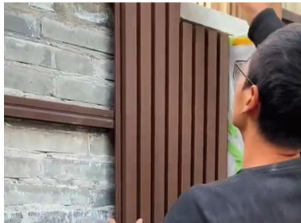
◦ Step 3 Arrange the products in a front-to-back order.
