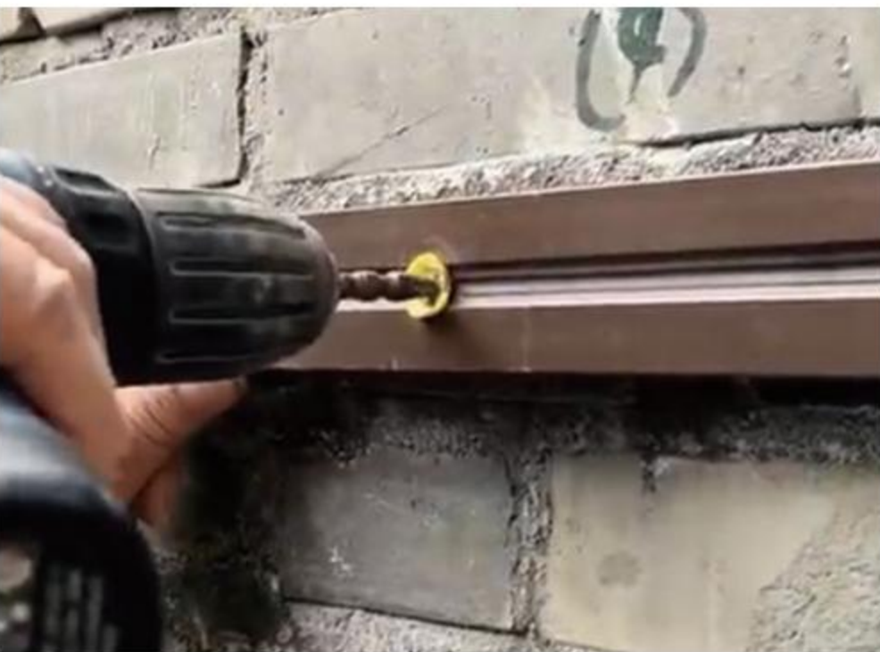
◦ Step 1 Fix the studs to the wall.
